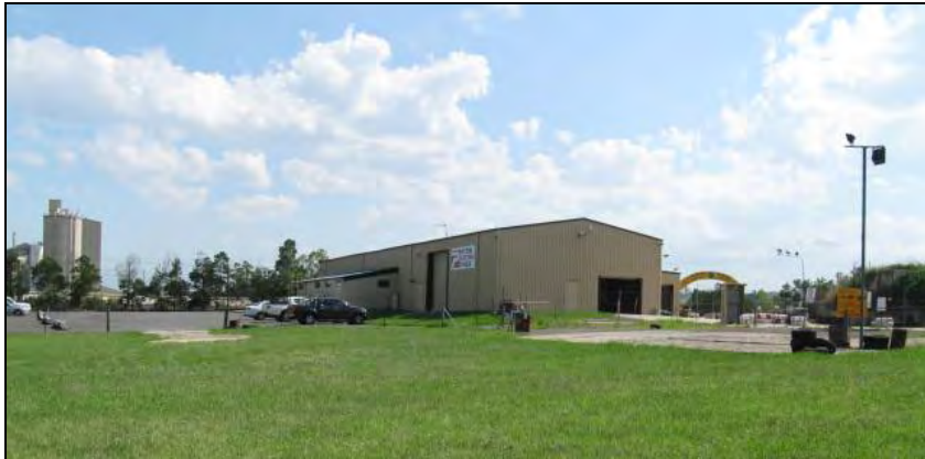
Plate 26: Existing commercial development – Go-Kart track and associated buildings, facing south east
