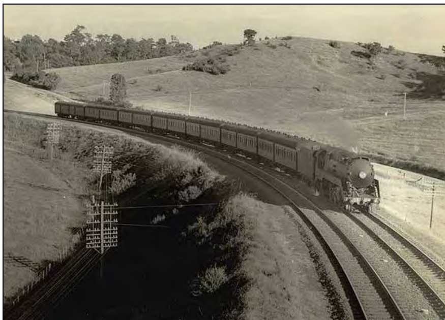
Plate 5 – 1955 image of C3804 'Melbourne Express' enroute through Maldon showing cleared land of the area and Razorback (Source: State Records -195517420_a014_a014000206).
